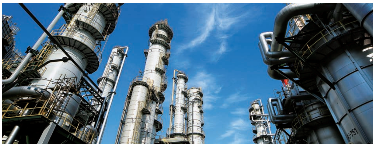
Kashima Oil Refinery's new petrochemical production facility
